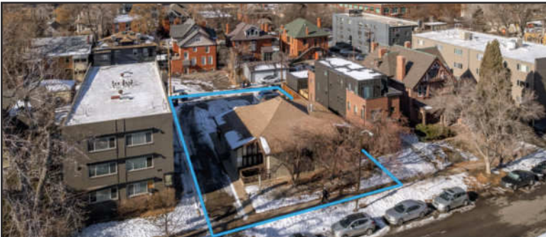
The former dental office was purchased by local developer McAtee Properties.
