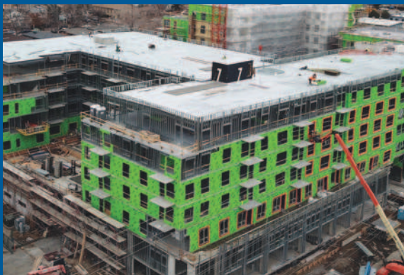
Zia Sunnyside (Under Construction)
