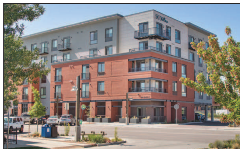
The 197-unit 281 Willow apartments is situated about a mile from the Colorado State University campus.
