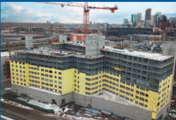
X-DEN (Under Construction)
