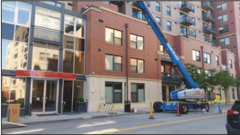
Making façade repairs can be a selling advantage.
