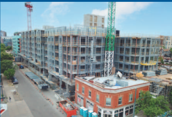
AMLI Uptown (Under Construction)
