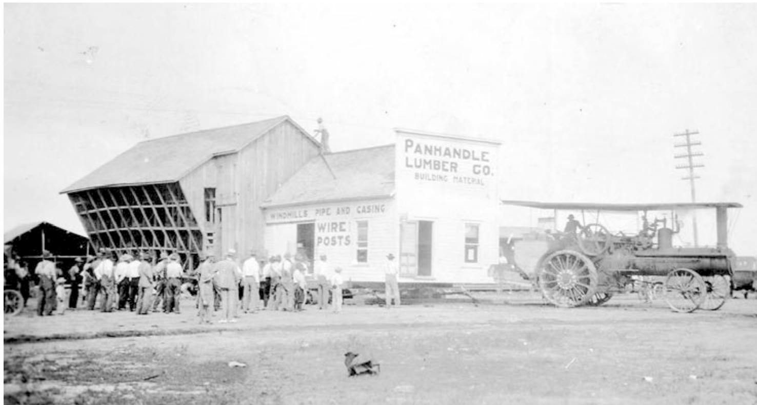
MOVING DAY — Huge steam powered tractors pulled building from Ochiltree, TX and Gray, OK to the new townsite of Perryton. Pictured is the Panhandle Lumber Co. building on its way to a new location in Perryton.
