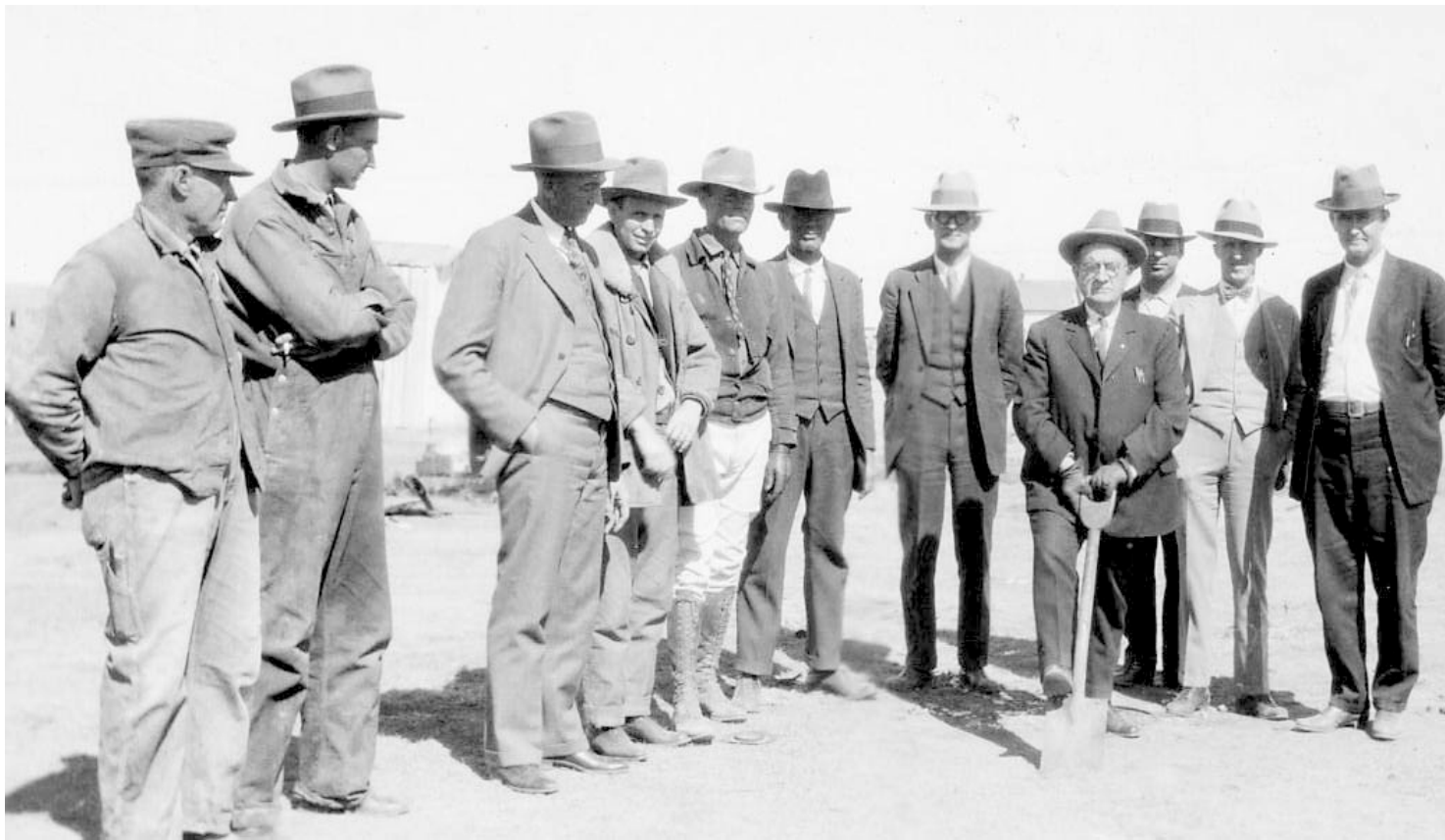
BREAKING GROUND — Ground was broken for the Ochiltree county courthouse in a ceremony in 1928 with Judge J.M. Grigsby at the shovel. Some of the other men are Sam Handy, H.C. Brillhart, W.G. Yeary, J.M. Bull.
