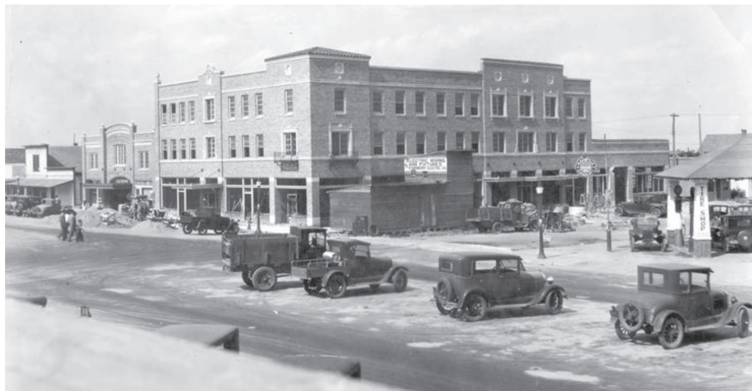
PERRYTON HOTEL — The pride of Perryton in 1929 was the new Perryton Hotel which is seen here under construction. At the left of the hotel is the new Ellis Theatre, another big construction project in that year of a bumper wheat crop and unlimited prosperity.
