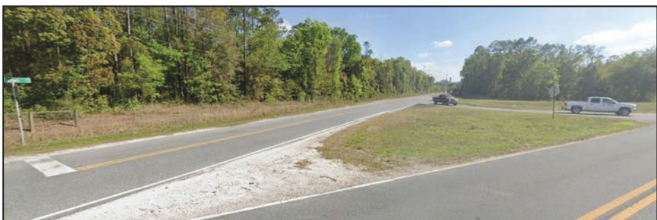
The work on Contractor’s Road, which has now entered the design phase, is the result of a partnership between Taylor County, the Florida Department of Transportation and Georgia-Pacific.
