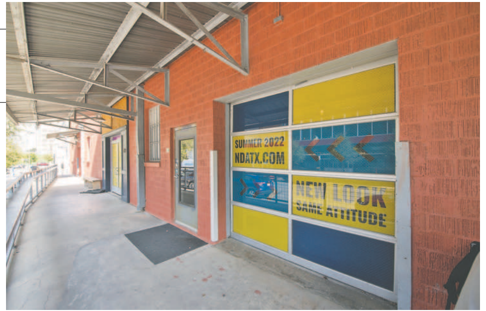
The new North Door at 908 E. Fifth, just 266 feet west of its former location
