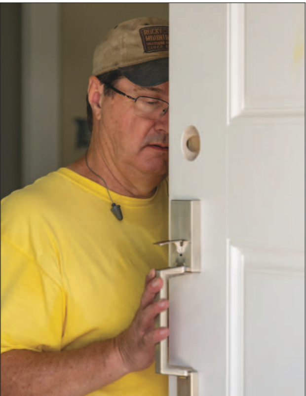
A volunteer installs the front door hardware.
