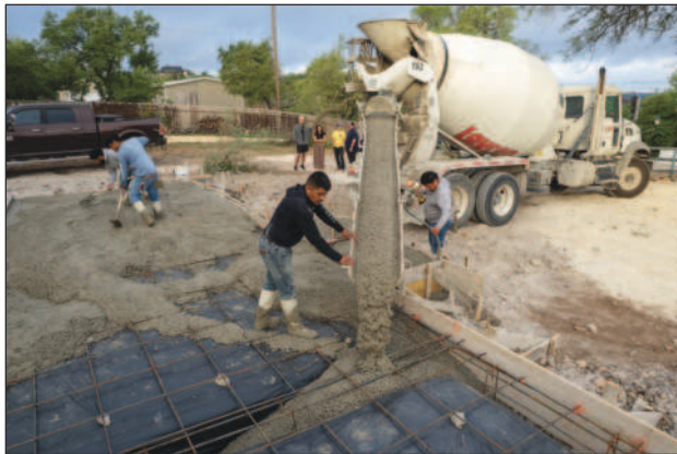
A crew lays the foundation.
