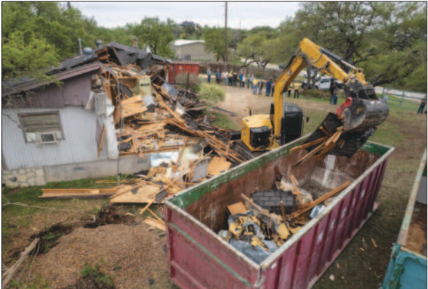
The McGoverns and the Hometown Missions team watch the house come down on demolition day.
