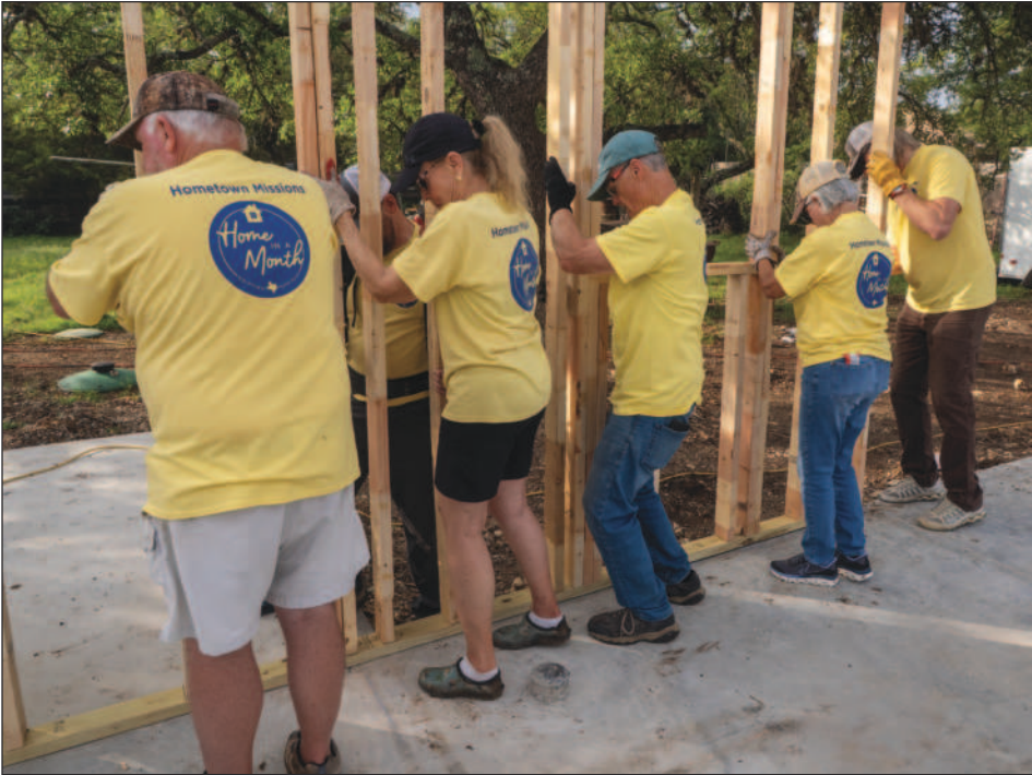
Volunteers get ready to secure a wall.
