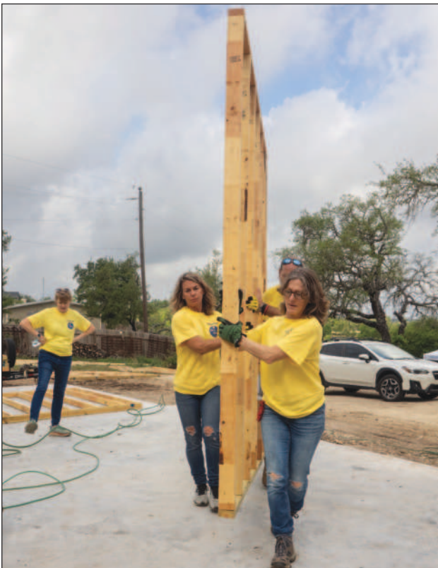
A team carries a wall into place.
