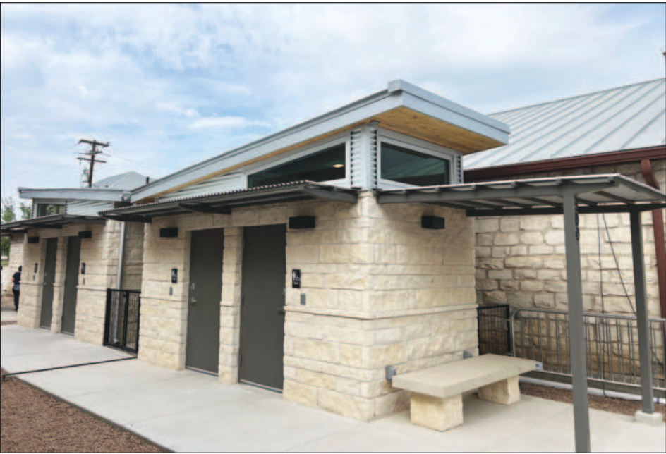
The restroom design fits into the style of the historical district.
