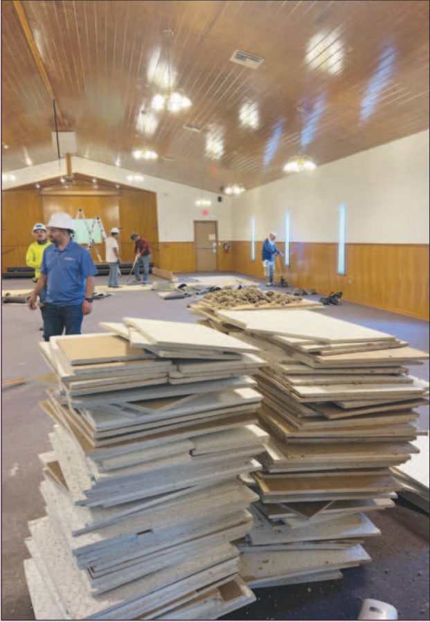
Contractors are already at work to remodel the City Hall building at 511 Mercer Street in downtown Dripping Springs. The $1.1 million project will add offices and upgrades to the building which houses administrative staff and is home to city council meetings. The project is expected to be completed by April 2025.
