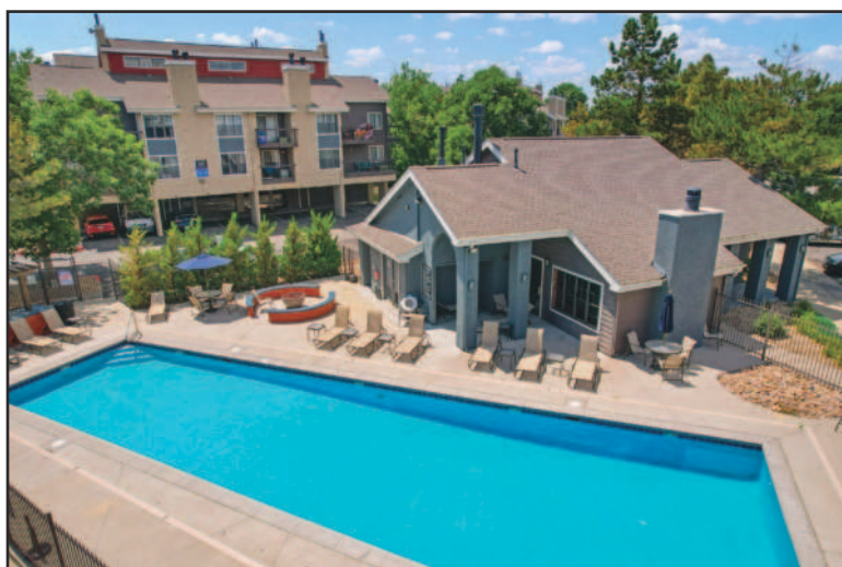
The 351-unit Advenir at Del Arte Apartments, located at 151 S. Joliet Circle, includes 17 buildings on 11.4 acres.
