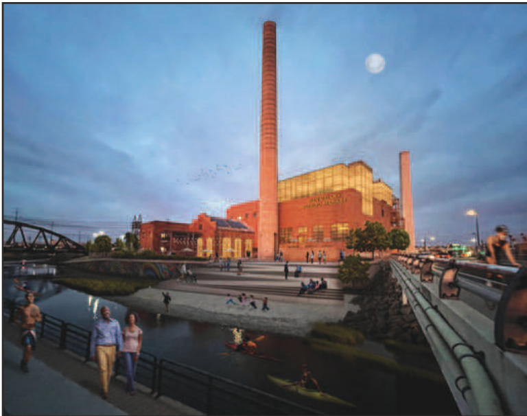
The Zuni steam power plant has been a continuous presence on the banks of the South Platte River for more than 122 years.
