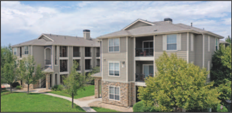
The Ridge at Lowry consists of eight, three-story buildings on 9.81 acres at 10000 E. Alameda Ave.
