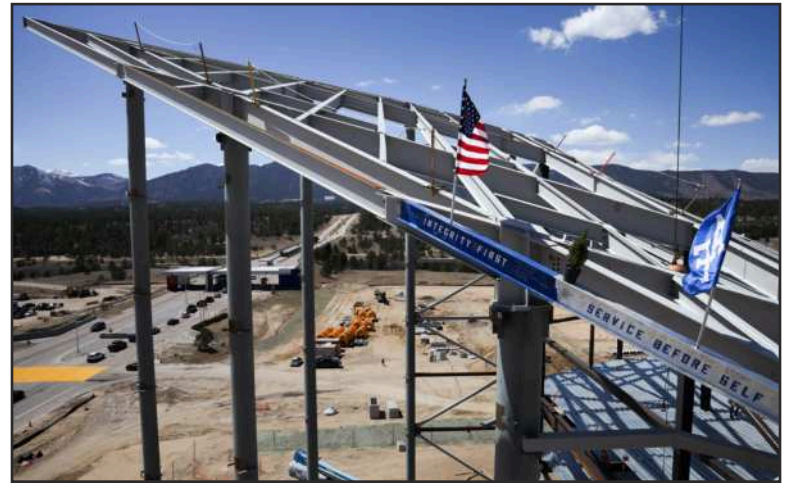
Construction crews topped off the 34,000-sf Air Force Academy Visitor Center.
