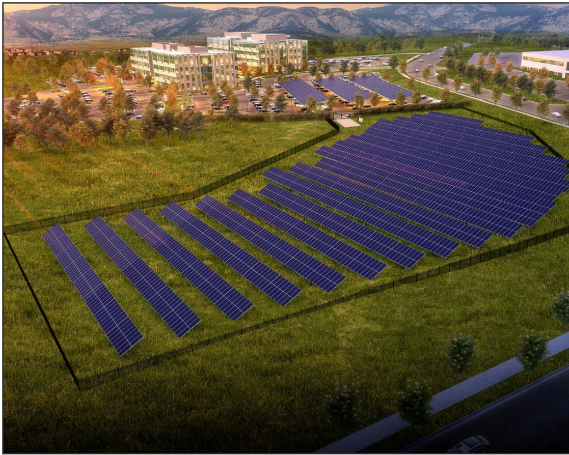
The solar installation will be one of the largest distributed solar projects in the city of Westminster.
