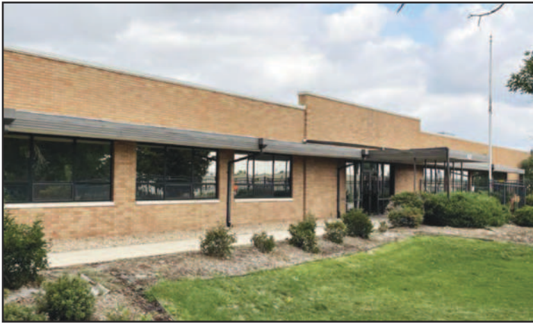
RFMX’s new industrial space is one of three locations in Colorado.
