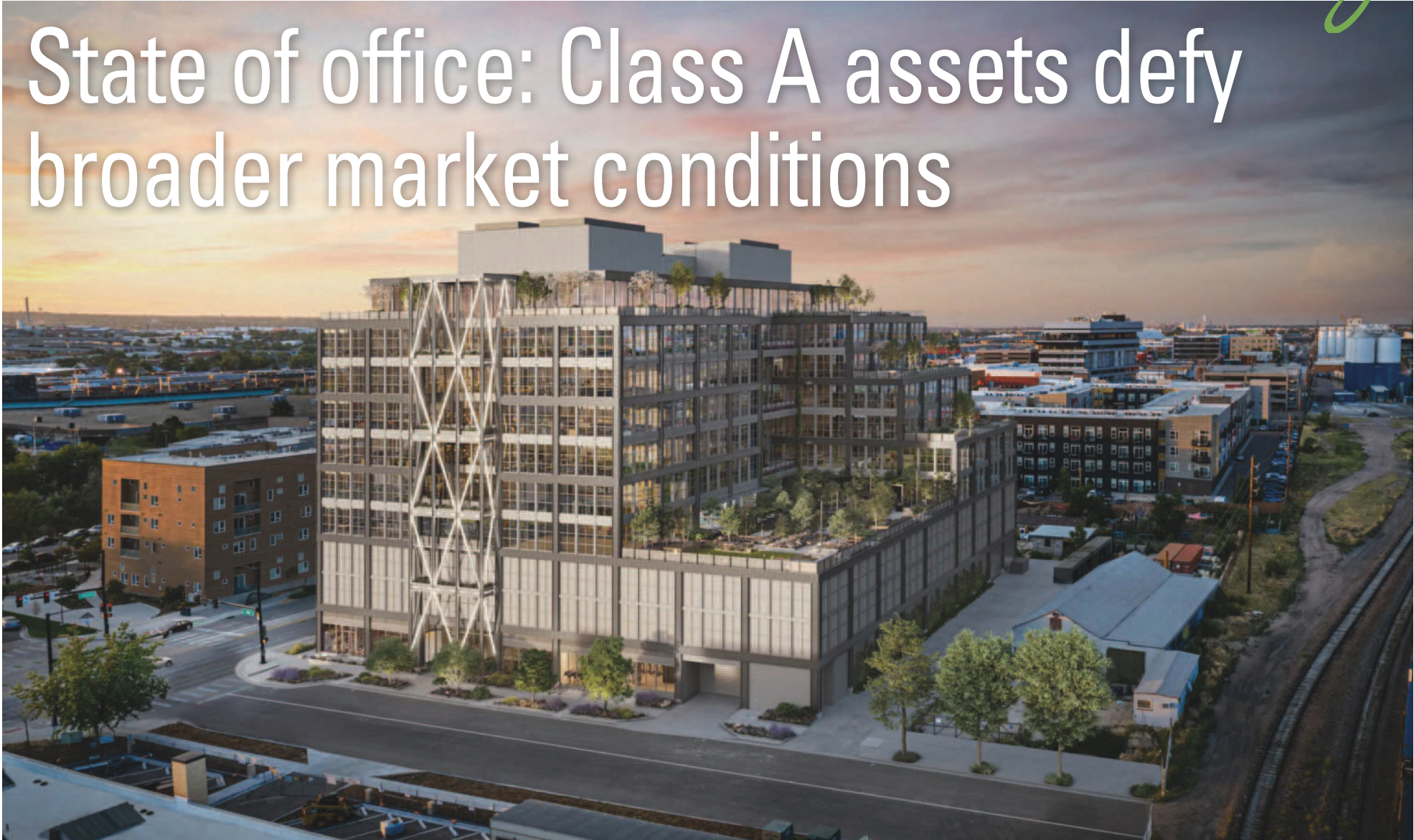
Steel House's industrial biophilic design, by Morris Adjmi and Open Studio Architecture, wraps around the largest elevated private park in RiNo.
