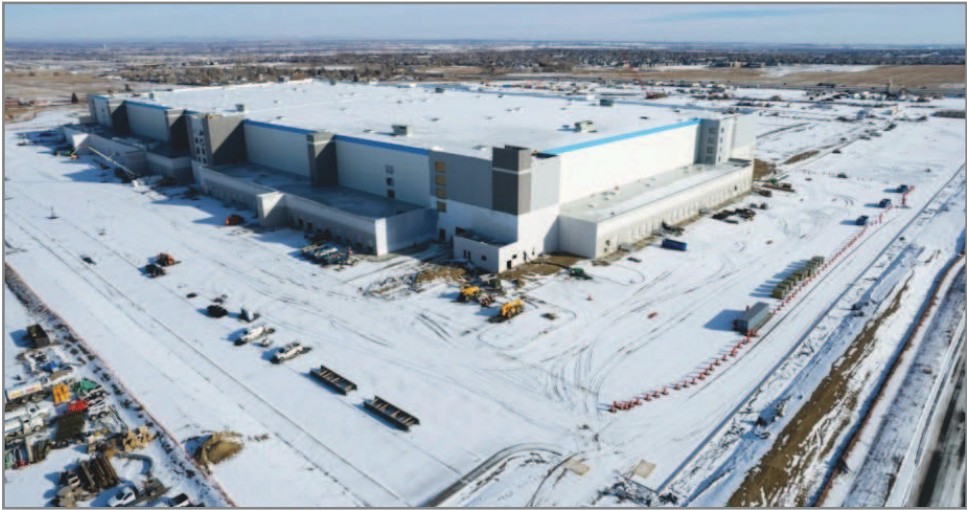
Amazon's new 3.9 million-square-foot facility under construction. Courtesy Trammell Crow Co.
