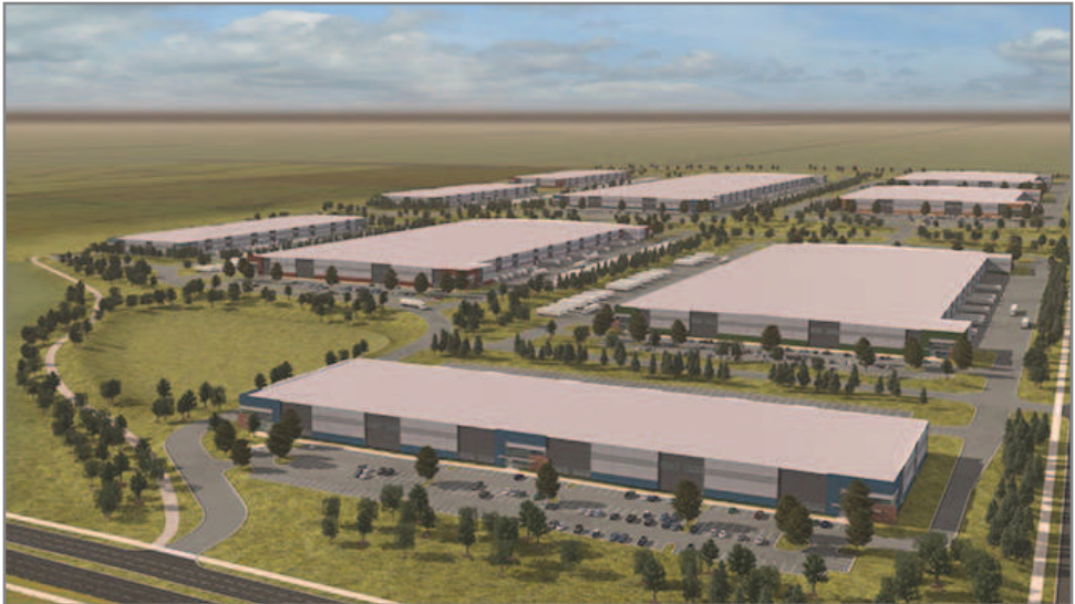
The first two buildings of Sun Empire – a 316-acre, 3.9 million-square-foot master planned industrial development – are underway in the airport submarket.
