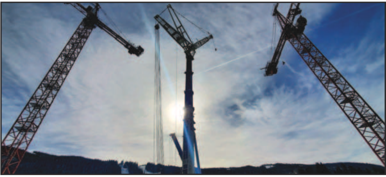
Kindred Resort is soaring upward with the recent installation of two tower cranes.
