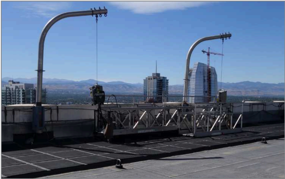
Approximately 30 years ago, a common davit arm installed on buildings was a curved, single-pole aluminum arm, also known as a "banana arm."
