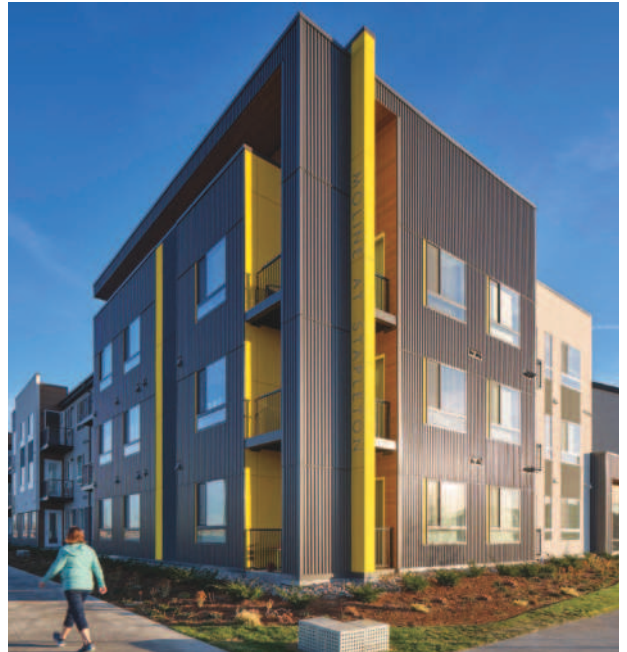
Ross Cooperthwaite Moline Apartments is arranged around a series of smaller, three-level, 12-unit clusters opening onto a common stair with warm wood stairs.
