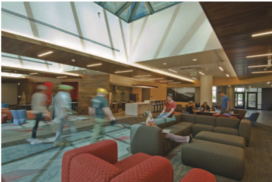
The lounge features skylights with electrochromic glazing that adjust their shading automatically based on the time of day and the season to save energy and reduce utility costs.
