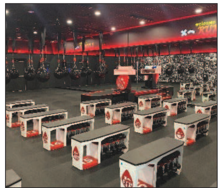
Sound dampening was a main concern for the adjacent tenants, so a rubber flooring system was installed throughout the space.
