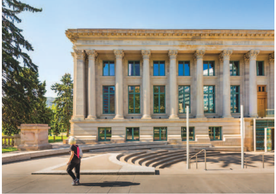
McNICHOLS CIVIC CENTER, DENVER, CO
