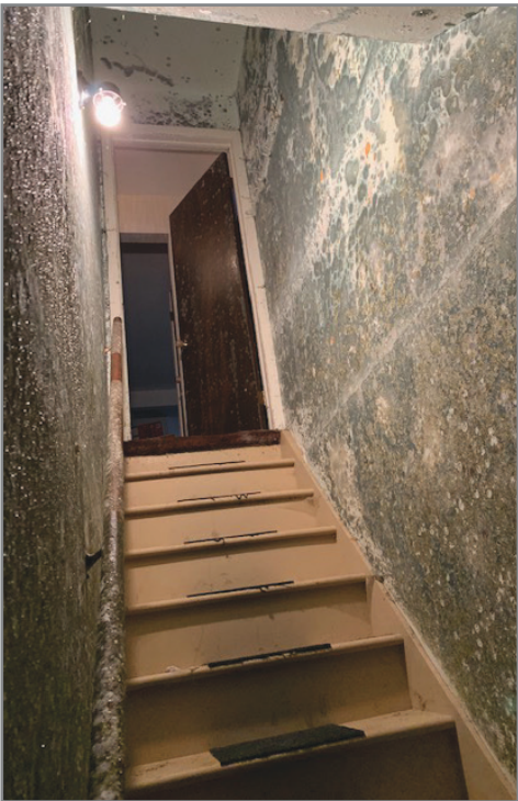
When mold spores fall on places where there is excessive moisture, such as where leakage may have occurred in roofs, pipes, walls, plant pots, or where there has been flooding, it will grow.
