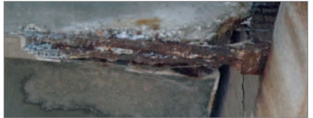
One common issue found is spalling of concrete due to corrosion of steel-embed plates, which often can be spotted at beam ledges, as water leaks through the joint above and sits on the ledge of the beam.
