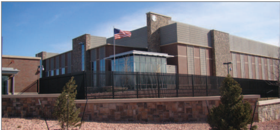
Often, data center exteriors include wall panels with a layer of insulation sandwiched between two layers of concrete. It is this construction method that generates the greatest thermal mass benefit of the enclosure system.
