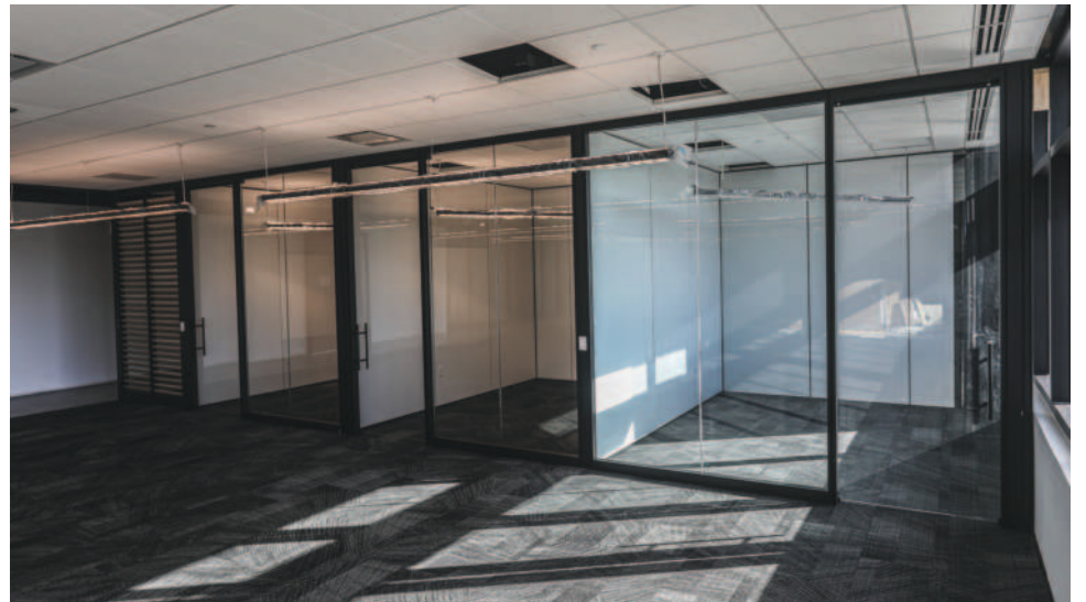
John Hoffman, Kiewit Corp. Office spaces can be reconfigured easily by using modular office wall systems like those pictured here inside Kiewit's regional headquarters in the city of Lone Tree.
