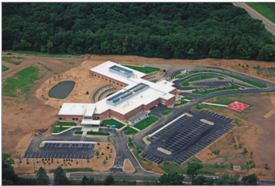
To minimize operating costs, this new construction rural hospital incorporated a geothermal system to achieve payback in less than five years.
