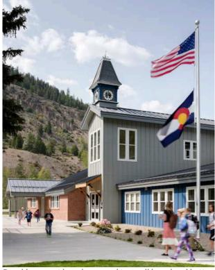
Durable cement board was used to recall board and batten siding, and the old school's exterior brick walls were left exposed to reflect the feel of the National Register Historic District in which the school is located.
