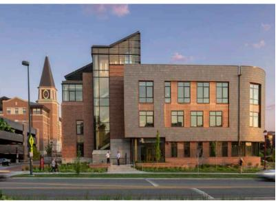
The exterior integrates traditional DU materials like red brick, limestone, sandstone, slate and copper.
