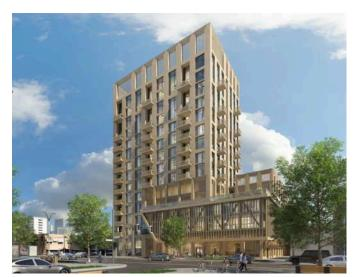
In response to the recent addition of new variations to Type IV construction in the International Building Code, KTGY's R+D concept, Timber Tower, proposes a 12-story residential design solution using cross-laminated timber as the primary structural material.
