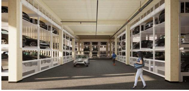
To maximize parking within a mass timber structure, mechanically stacked parking fills a single-level garage at the ground floor of Timber Tower.
