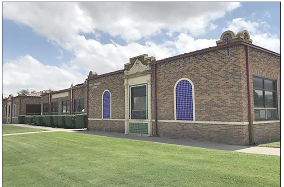
Alpine ISD Administration Building
