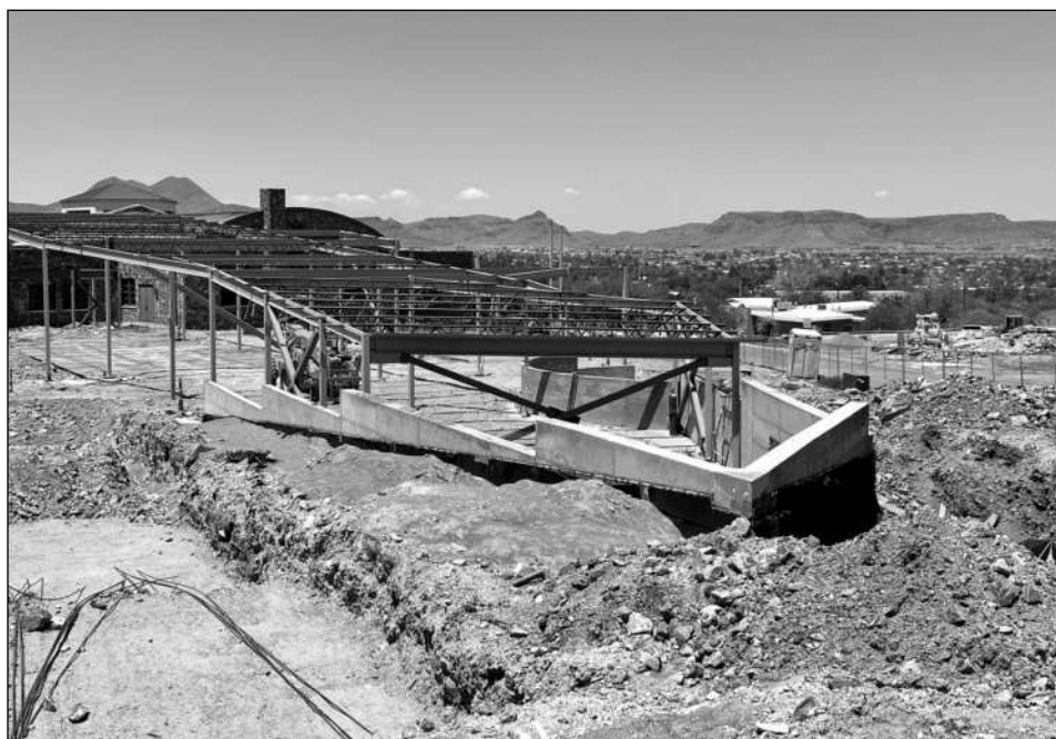
Expansion is in progress at Museum of the Big Bend.
