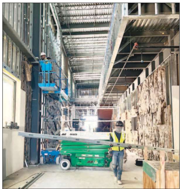
Construction continues at the new Alpine High School.
