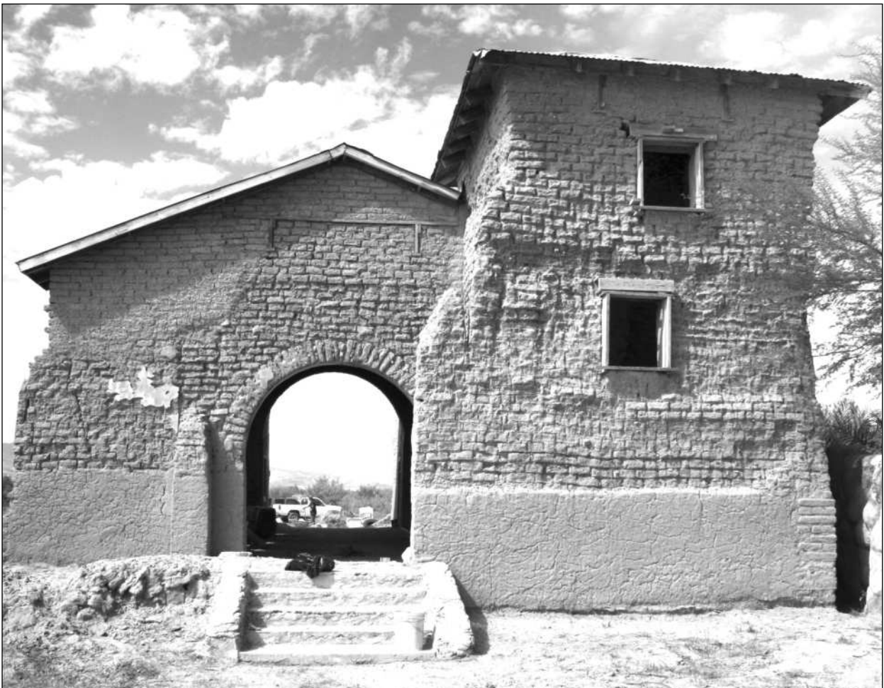
On Saturday, Oct. 23, from 11 a.m.-4 p.m., Friends of the Ruidosa Church will host an open house at the recently restored building in Ruidosa on FM 170 west of Presidio. The church was built in 1915, but fell into disrepair, and by 2000 the Diocese of El Paso recommended it be torn down. In 2019 it was turned over from Presidio County to the non-profit Friends group for restoration and repair.
