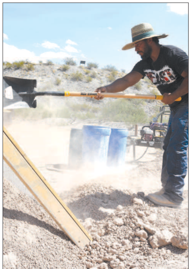
Sifting clay is part of the prep work at the site of the Alvino House preservation project in Big Bend National Park.
