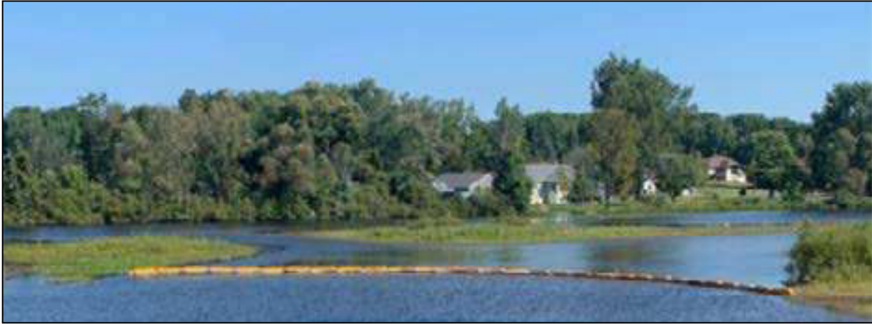
Turbidity curtains will contain excess silt while Lake Shamrock is dredged
