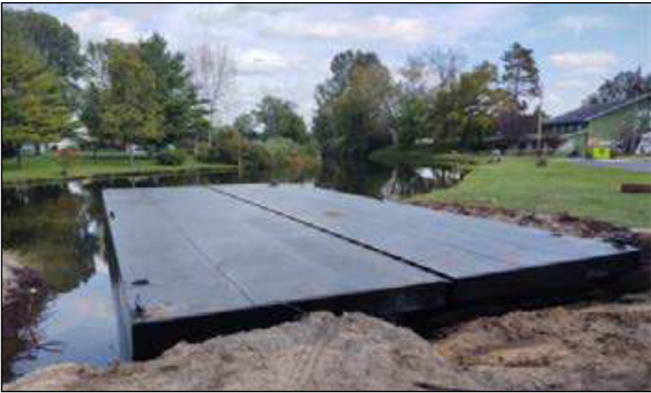
The barge for the silt material to be dredged from Lake Shamrock, is together and ready for dredged material.
