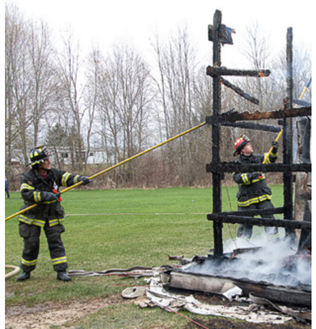
Firefighter Jim Doherty and Lt. Tracy Pohl were pulling apart the barn structure that remained standing after the blaze was extinguished.
