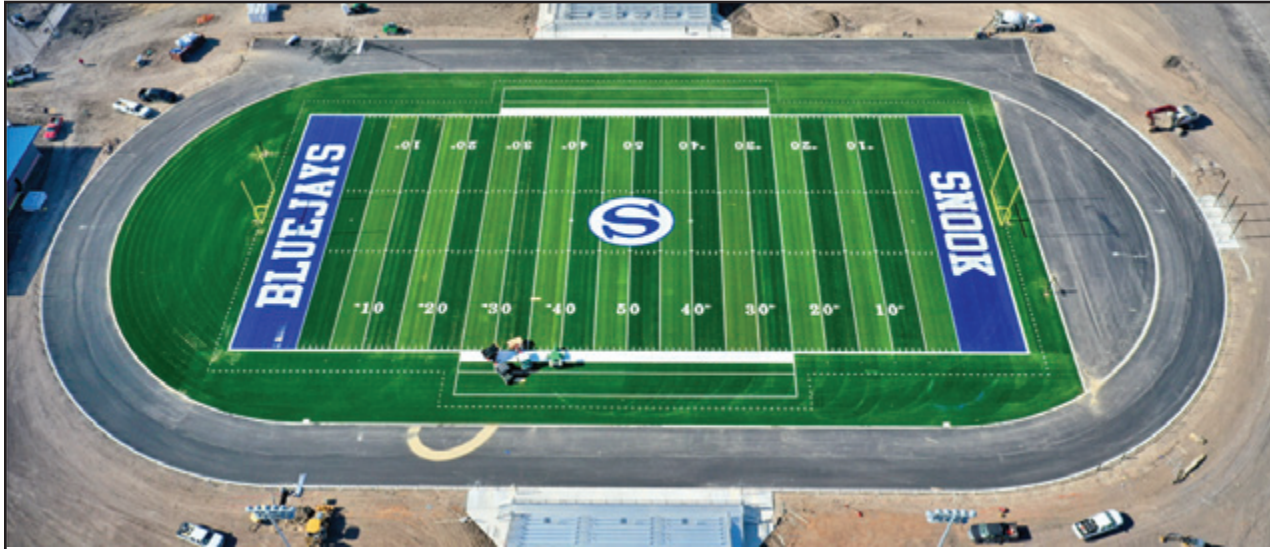
THE TURF HAS BEEN PUT IN PLACE, and the rubber track surface is currently being installed at the new Bluejays Stadium at Snook Secondary School. This project is part of the voter approved bond for a multipurpose athletic facility. -- Drone photo courtesy of Snook ISD
