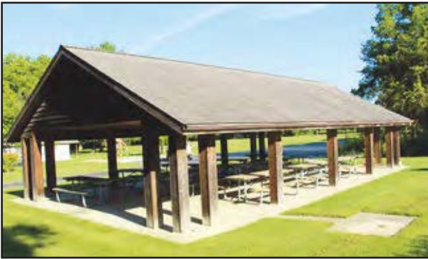
This pavilion at William Henry Harrison Park attracts picnic goers and is one of several in the park district.
