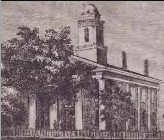
Wood County Courthouse, built 1843.
