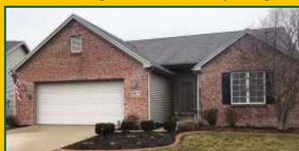
10172 N. Shannon Hills Drive, Perrysburg
