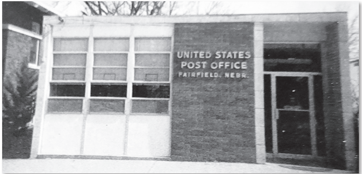
Fairfield Post Office.
