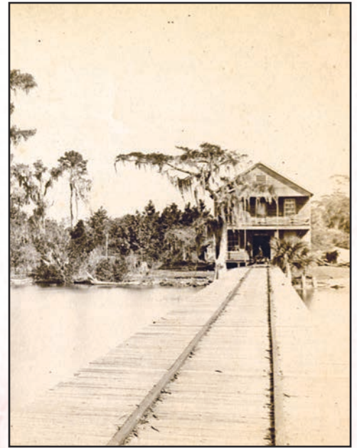
A general store on the lake at Georgetown. The dock was equipped with a track to load and unload fruit and supplies from the ships that made their way up the St. Johns River.
