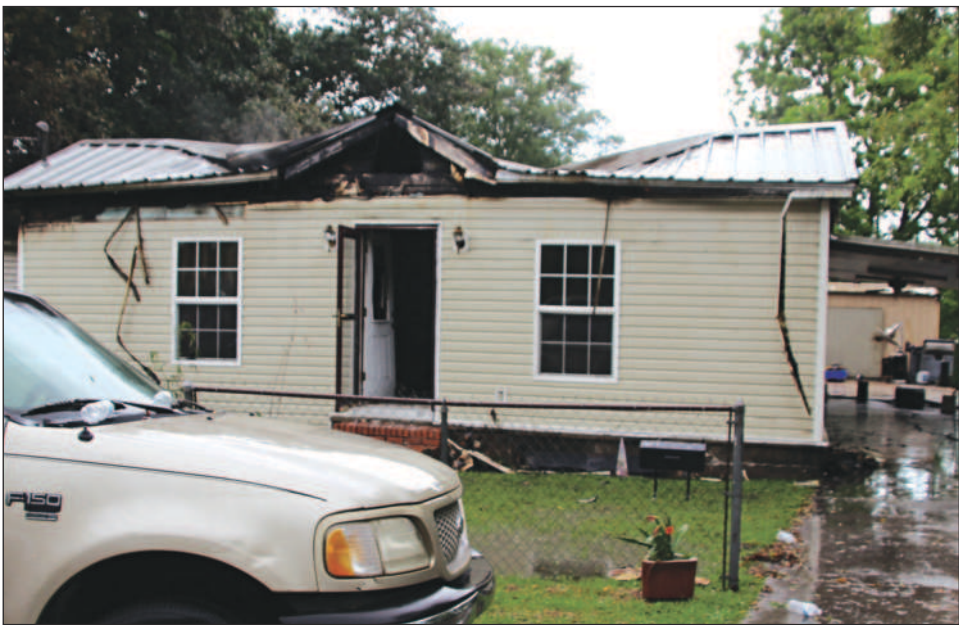
A fire on Monday destroyed a house at 710 Tate St. (Photo by Myra Miller)
