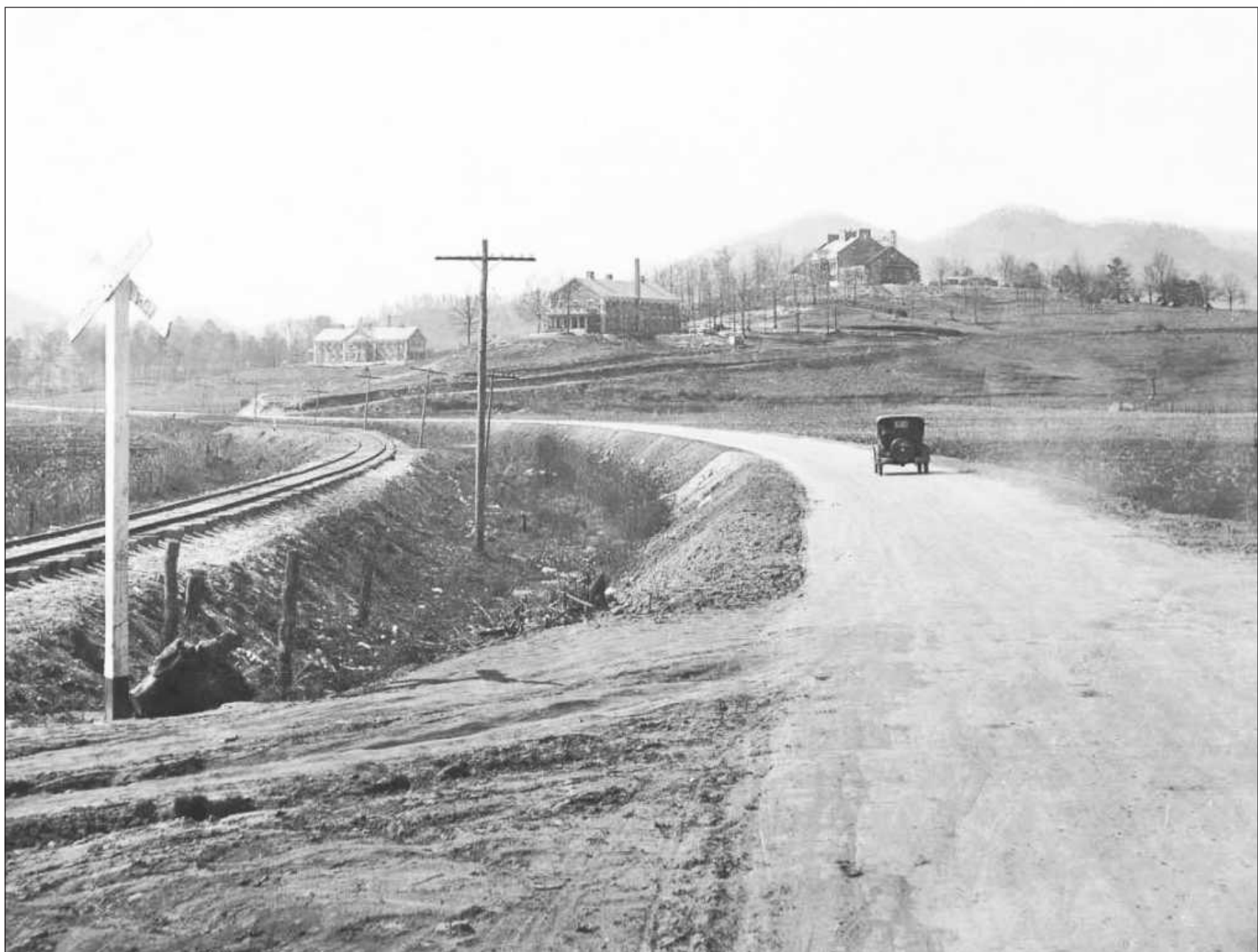
In April of 1928 the main north-south highway had just been hard-surfaced with crushed granite. The Tallulah Falls Railroad can be seen on the left and the newly rebuilt, after a fire, Rabun Gap-Nacoochee School in the background.
