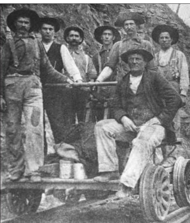
Tallulah Falls Railroad construction workers are pictured circa 1900.
