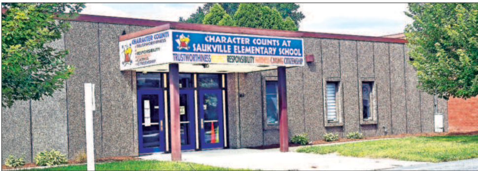
BUILT MORE THAN 70 years ago, Saukville Elementary School is in need of significant work. A Port Washington-Saukville School District plan that is the subject of a survey to be mailed to residents next week calls for replacing it with a new school on a new site. Press file photo
