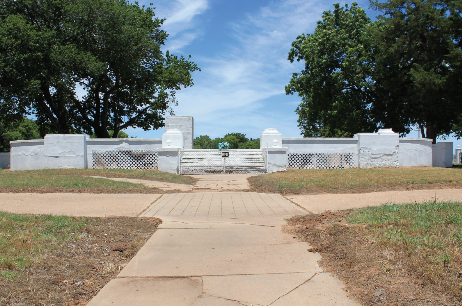
The once grand 101 Ranch White House was leveled to the foundation in 1943. (Photo by Laci Jones)
