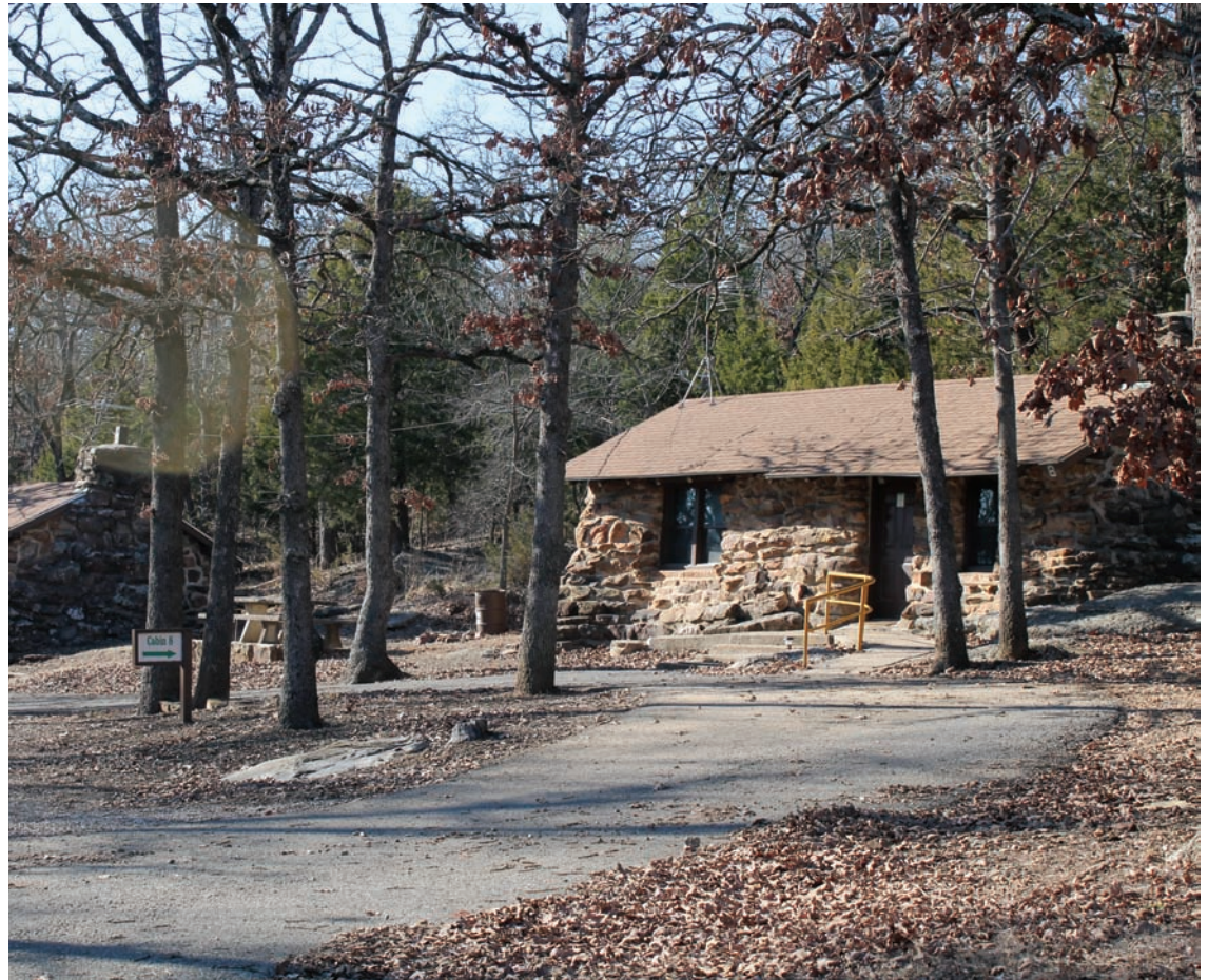
The WPA crew built ten native stone and wood frame cabins. Five other rock veneer cabins were built at a later date. (Photo by Laci Jones)
