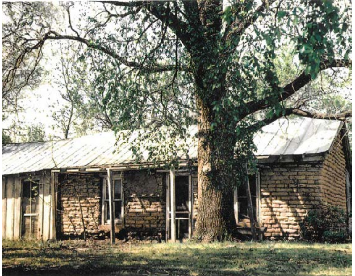
The oldest house in Wilbarger County is an adobe at Doans, the 1881 home of Corwin F. Doan, who operated a trading post nearby that served trail drivers, Indians and early-day settlers. The picture shows the landmark adobe as it appeared in the early 1990s before a 1993 restoration resulted in the removal of the frame addition and the addition of an EIFS (Exterior Insulation Finishing System, essentially synthetic stucco) sheathing that changed the exterior appearance. (Photo by Hanaba Welch)
