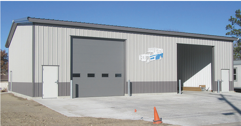
NEW AMBULANCE GARAGE is nearing completion southeast of Boone County health Center.
