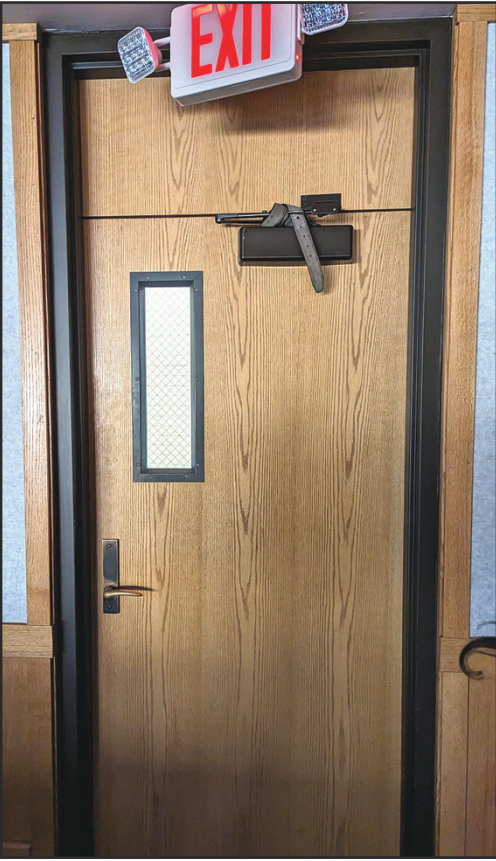
PHOTOS such as this of a belt used to try to keep doors from being opened were circulated last week by law school students upset that some classroom doors could not be locked. (Winni Zhang photo)
