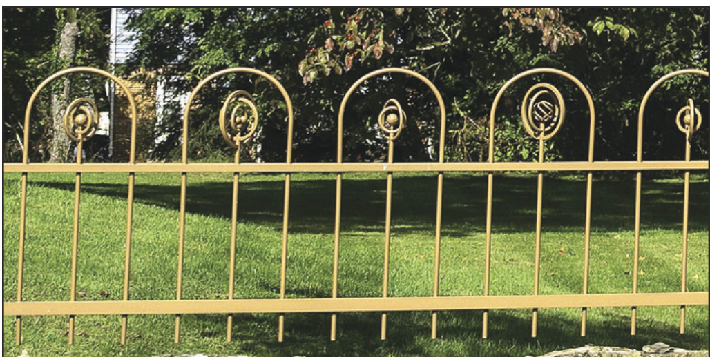
THIS Communion of Saints Railing outside of Good Shepherd Evangelical Lutheran Church was completed and installed last year and dedicated this month.
