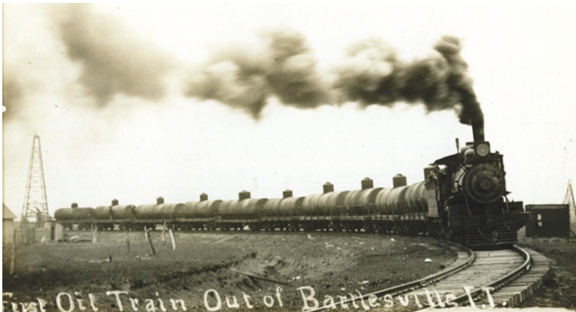
This is the first oil train leaving Bartlesville with a load of unrefined oil.
