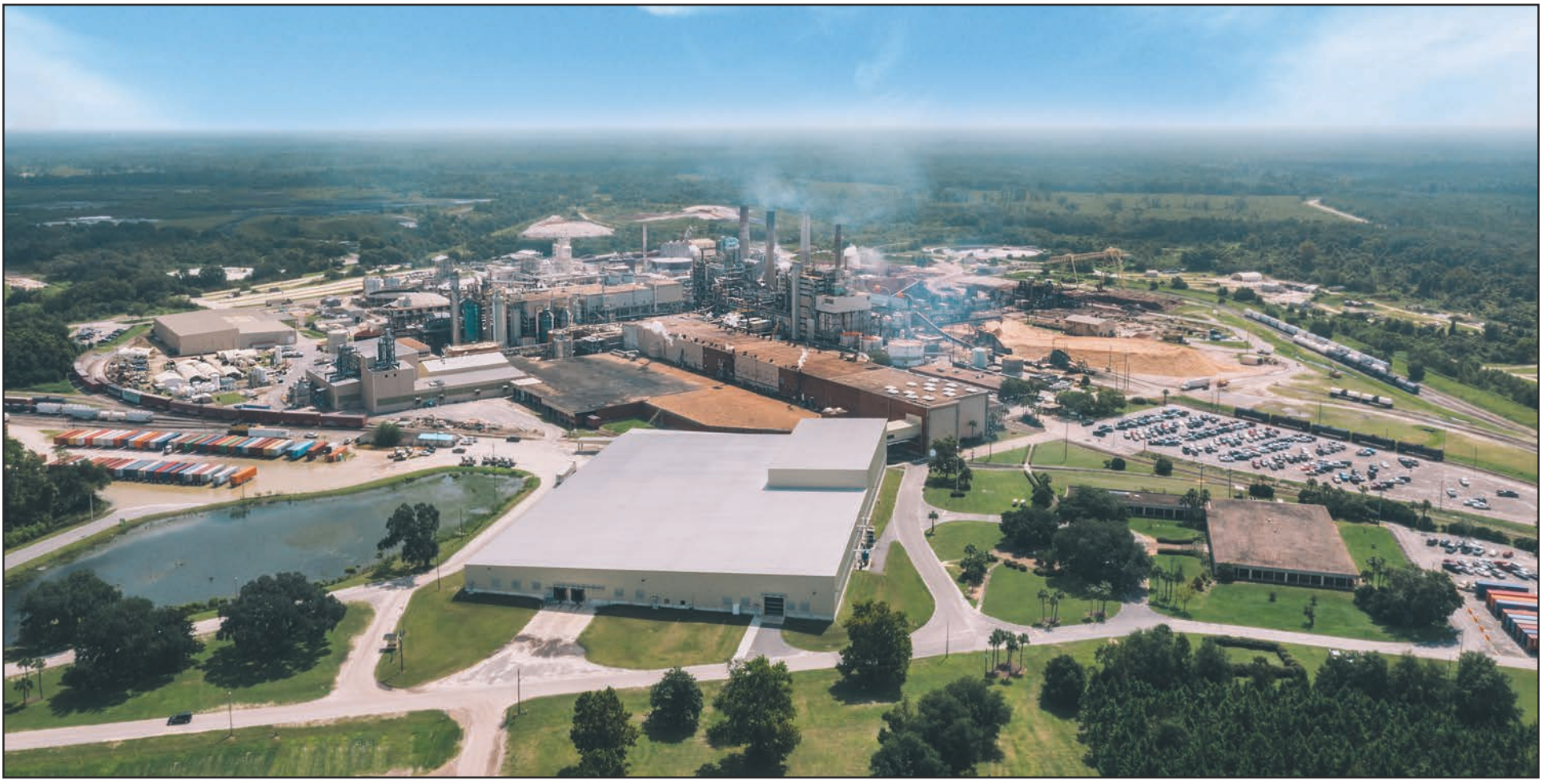
The local Georgia-Pacific (GP) Foley Cellulose mill has returned to full operation and is now undertaking a new $30 million investment project in 2022.
