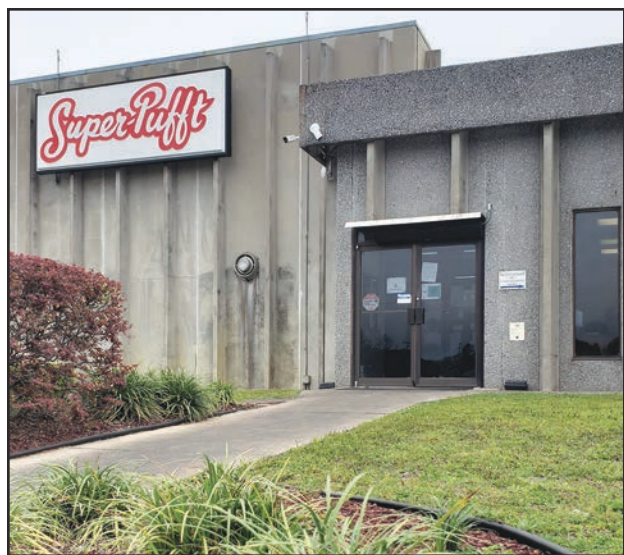
A workforce of approximately 300 employees keep the lines running nearly 24 hours a day.
