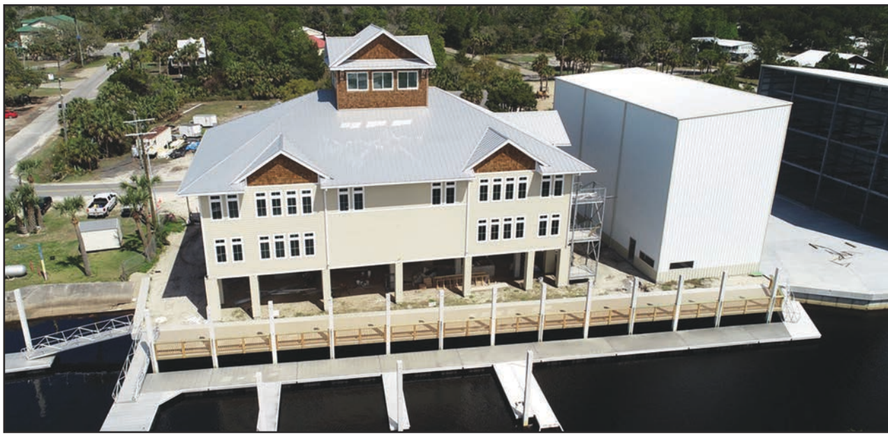
Steinhatchee Marina at Deadman's Bay will feature a three-story marina building containing multiple uses (including a tavern), dry-stack boat storage for up to 48 vessels and 82 wet slips.
